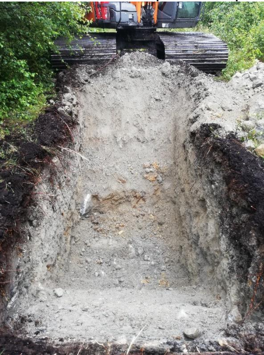
Plate 34: TPCC4 alternative trial pit excavated.
