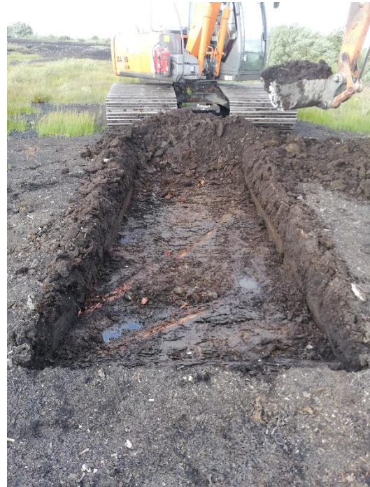
Plate 28: TPCC2 showing wood therein.
